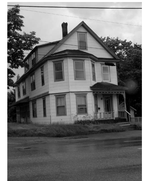
House on Katahdin Avenue
